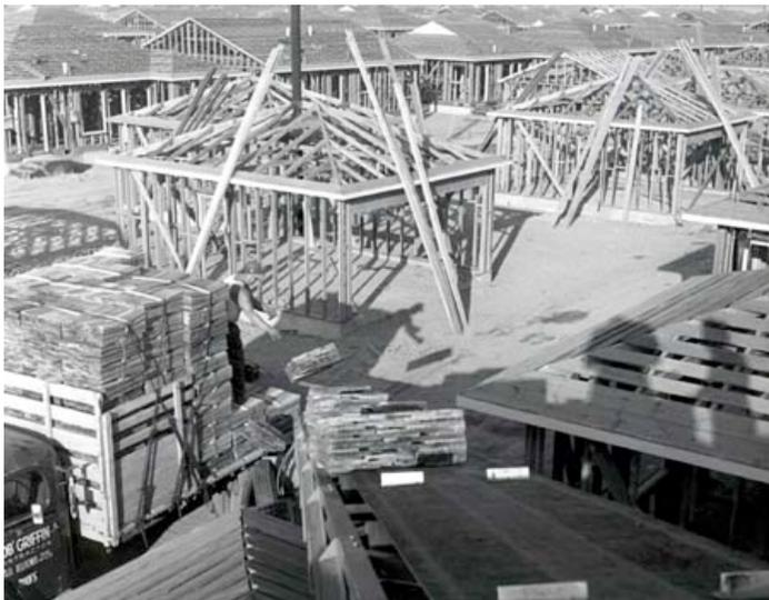
*The construction of Lakewood Subdivision - note the conveyor belt to bring tiles to roof. Image courtesy of the City of Lakewood.*
